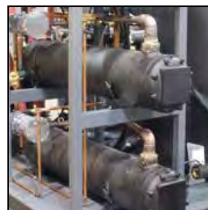
Water-cooled condenser. Configuration may be different on specific units.
