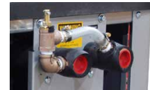
Typical optional automatic low flow bypass valve.
