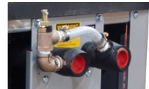
Typical optional automatic low flow bypass valve.
