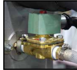
Optional Make-up solenoid valve (typical).
