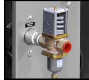
Typical water saver regulator valve.
