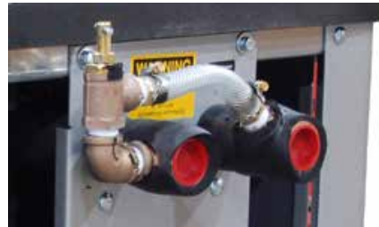
Typical Automatic Low Flow Bypass Valve
